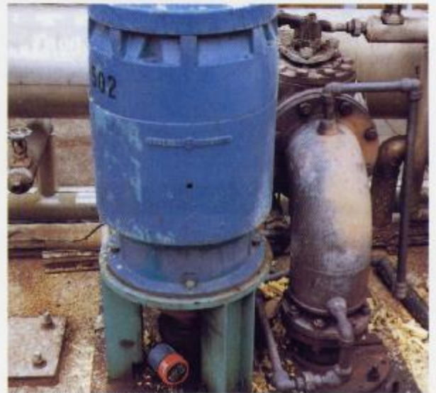
PUMPING STATION — U.S.A.
